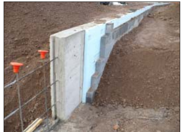
Figure 2 - Rigid Vertical Foundation Insulation
