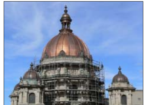
Onondaga County Courthouse dome restoration in progress
