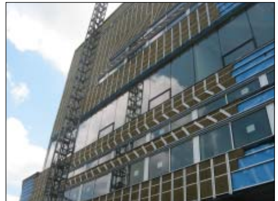
The Center of Excellence Rain Screen Facade
