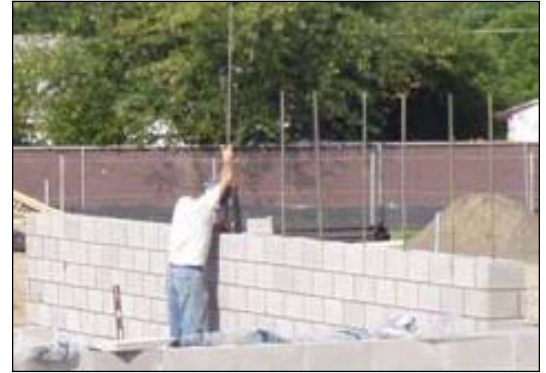
Threading rebar positioners for low-lift grouting
