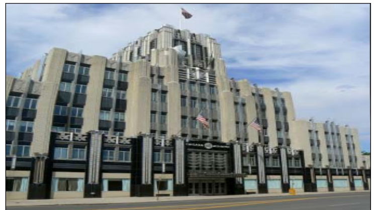
The NiMo Building, constructed in 1932
