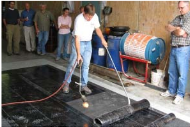
Jamie Trevvett, left, practices an application of torch applied roofing during the Roofing Workshop at the Henderson Johnson facility on Canal Street in Syracuse. Watching him at right is Richard Colson, a project manager at Bell & Spina Architects. Below, Janice Medina, Jamie Trevvett and Neil Garry, P.E., apply liquid roofing onto reinforcing felts on a roofing mockup.
