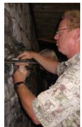
Janice Medina, left, shows an area of wall to which she applied mortar during the Masonry Workshop in Skaneateles Falls. Rich Applebaum, right, carefully practices his pointing skills with the natural cement.
