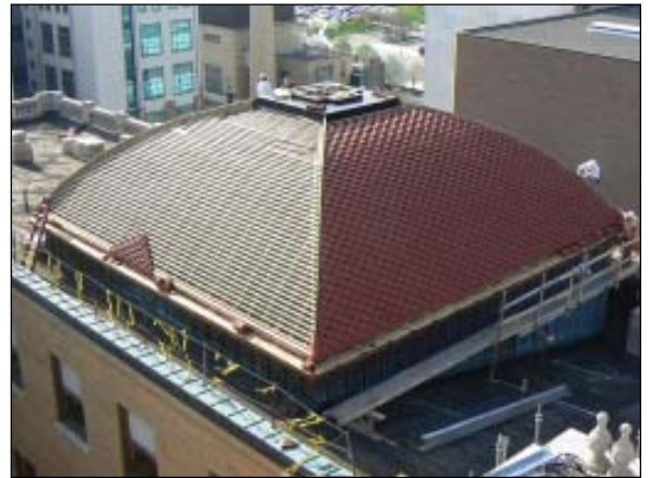
An upper view of one of the Onondaga County Court House domes, with the tile in place on one side and the wood lath visible on the adjoining plane. Below left, workmen proceed on the tile work, with the modified bitumen protective covering of the main dome visible in the background.
