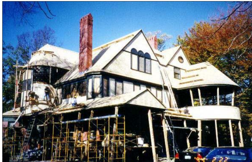
Isaac Bell House - Renovation
